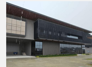
Malaysia Operations Center (being constructed)
