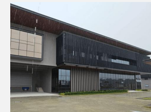
Iskandar Puteri, Malaysia Operations Center (being constructed)
