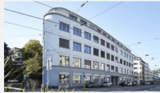
Zurich, Switzerland R&D Office
