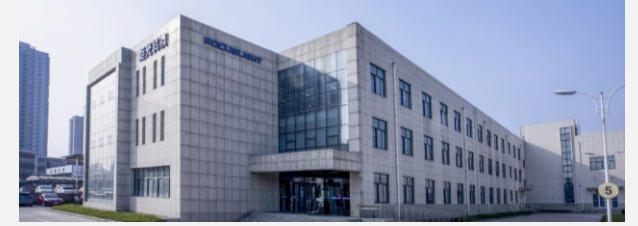
Xi'an, China Focuslight HQ, Operations Center
