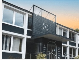
Neuchâtel, Switzerland Operations Center
