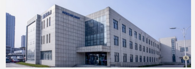
Xi'an, China Focuslight HQ, Operations Center
