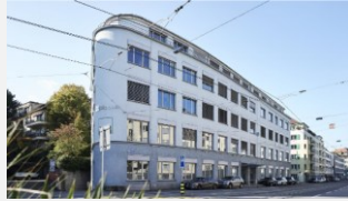
Zurich, Switzerland R&D Office
