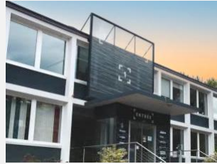
Neuchâtel, Switzerland Operations Center
