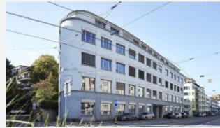
Zurich, Switzerland R&D Office
