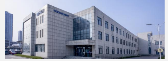
Xi'an, China Focuslight HQ, Operations Center
