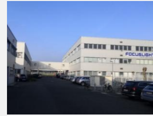
Dortmund, Germany Operation Center
