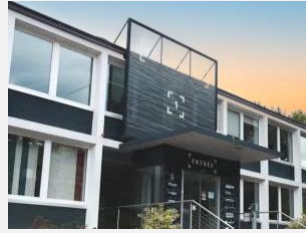
Neuchâtel, Switzerland Operation Center
