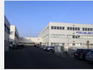
Dortmund, Germany Operation Center
