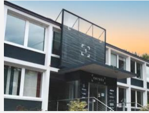
Neuchâtel, Switzerland Operation Center
