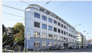
Zurich, Switzerland R&D Office
